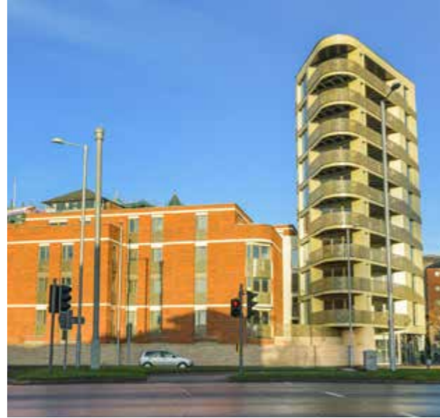
HyLyfe - 92 BTR Apartments. London Road.
