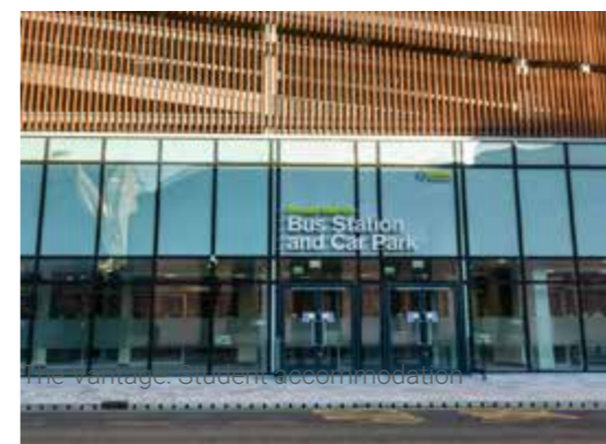
The new Broadmarsh Bus Station and Car Park. Canal Street.
