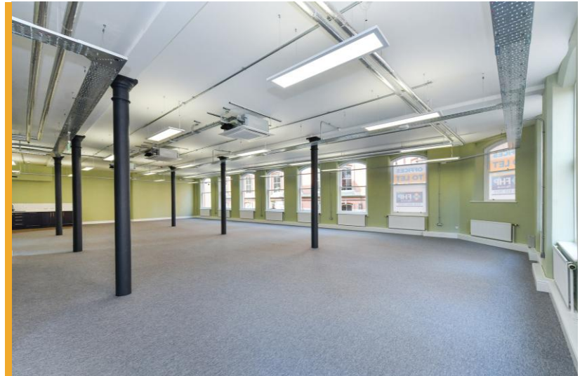
Images of the recent refurbishment carried out on the first floor.
