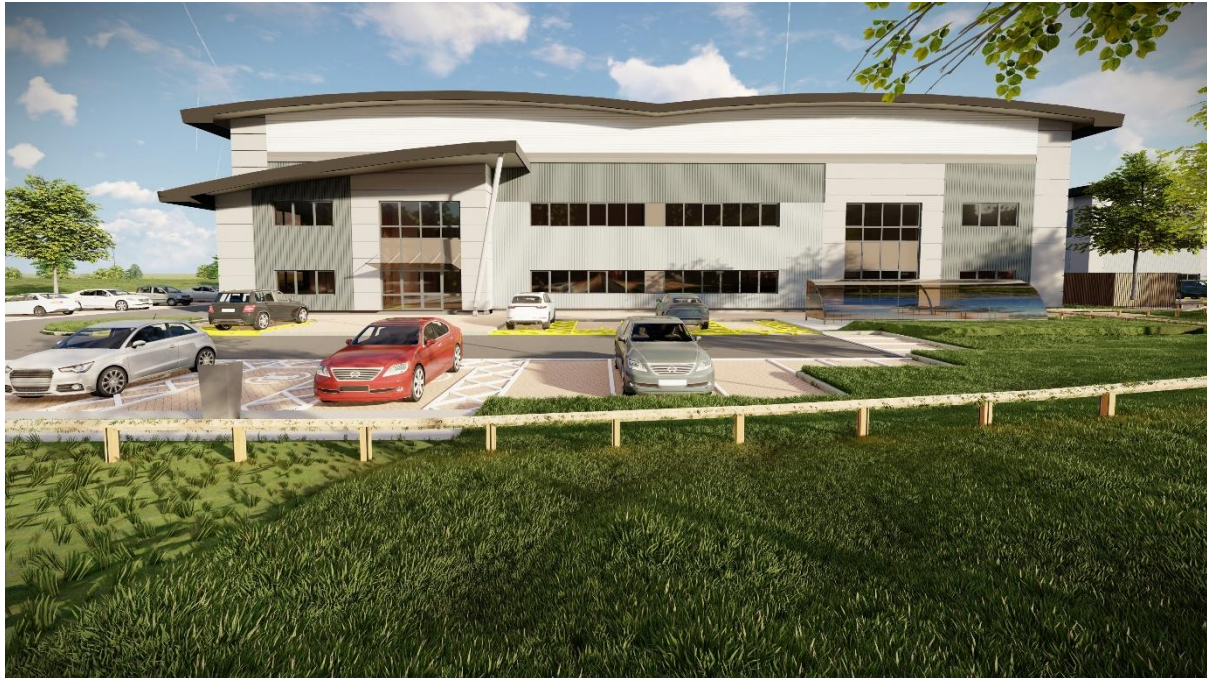
[Phase Two Unit D1 - Fairham Business Park]
